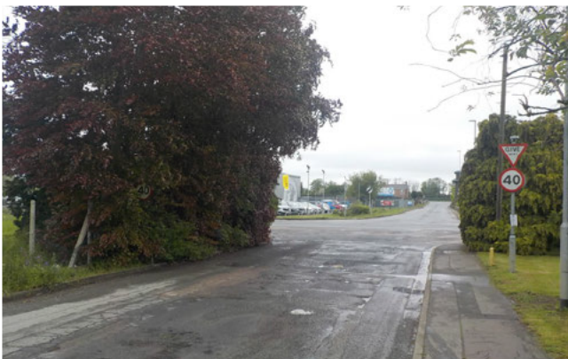
Figure 9 – View looking west on New Bridge Lane (East) at Cromwell Road junction.
